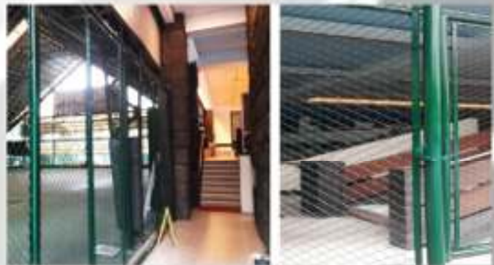
Repair of Indoor and Outdoor Court Fences
