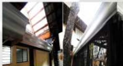
Repair of Log Cabin Gutter
