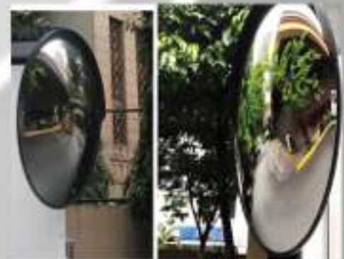
Installation of Convex Mirror
